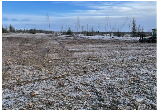
These photos show the work on the first pass in the winter/spring of 2023 / 2024, shredding the residual wood after logging. This was not yet incorporated into the ground. This was a 270 hp hydrostatic mulcher and it took 4 to 5 hours per acre.
